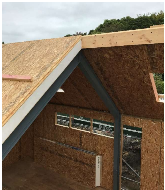
3 - Formance roof panels complete the envelope
